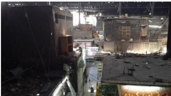
Figure 16. The deteriorating first floor and overlooking the random expansions done by tenants.
