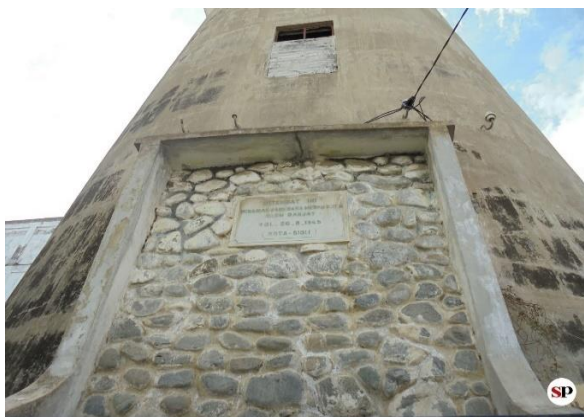
Gambar 2. Tower Air Belanda Block Bengkel (Ula, 2017)
