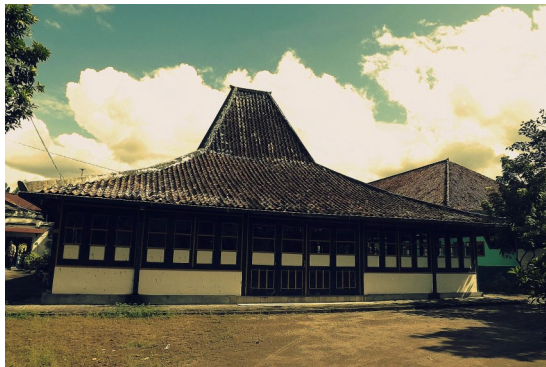
Figure 2. Kyai Pengulu's residence in Kauman Village Yogyakarta [18]
