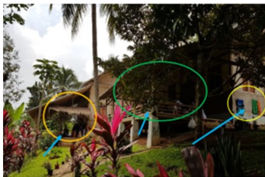
Figure 3. Al-Ischakiyah Islamic Boarding School (Existing)
