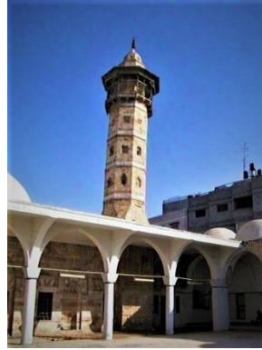
Figure 11. Gallery at The End of The Shaft, Sayed Hashim Mosque, Gaza, Palestine (Source: Iwan Center for Heritage Architecture, Islamic University Gaza, Palestine)
