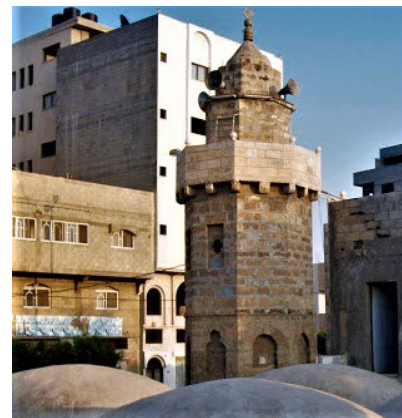
Figure 3. The short minaret of Ibn Marwan Mosque, Gaza, Palestine (Source: Iwan Center for Heritage Architecture, Islamic University Gaza, Palestine)
