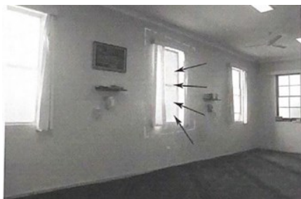
Figure 14. The windows, especially in the main prayer hall are highly recommended to be replaced with glare-reducing glass to overcome the long hot evening sun during summer.
