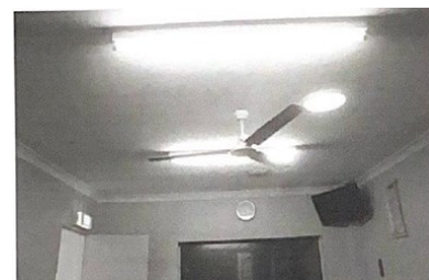
Figure 20. The current ordinary lighting fixture in the female prayer room, to some degree, brings out the glare experience to the users.
