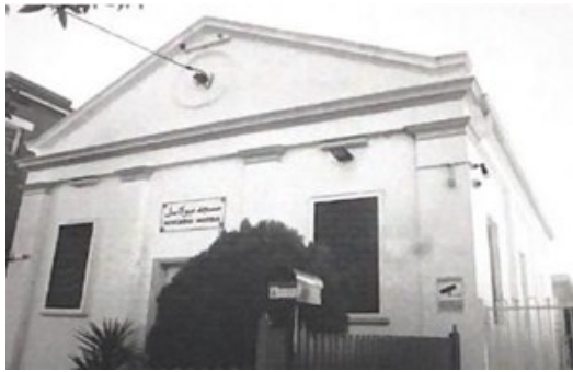
Figure 1. Newcastle Mosque in Newcastle, New South Wales, Australia
