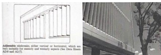
Figure 11. Adjustable sunbreak, either vertical or horizontal, which are very suitable for easterly and westerly aspects
