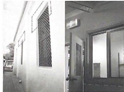
Figure 16. The designated windows at the Newcastle mosque should be highly suggested with blinds and awning on the exterior
