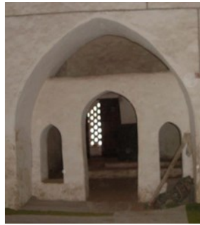
Figure 18: Entrance of the mausoleum from section (C) south.
