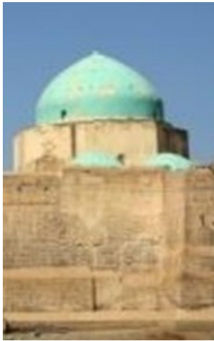
Figure 49: Octogon drum of dome school of Al-Iskandariyah [14]
