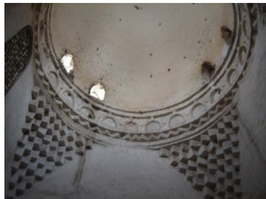
Figure 16. Triangle pendentives of Mustafa Pasha's mausoleum dome in Zabid (Author's photo 2014).
