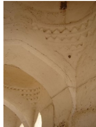
Figure 21: transition zones of Domes of the portico (triangles stalactites) (Author's photo 2014).
