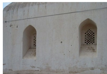
Figure 7: Shapes of three-pointed arched windows of The Madrasa of Mustafa pasha in Zabid from the northern façade (Author's photo 2014).
