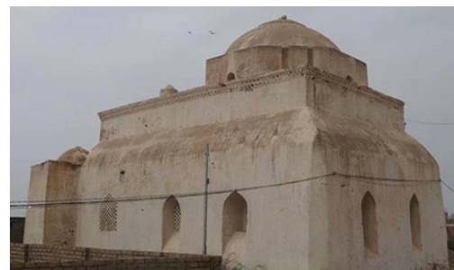
Figure 6: Abutment walls that supported walls of The Madrasa of Mustafa pasha in Zabid (Author's photo 2014).
