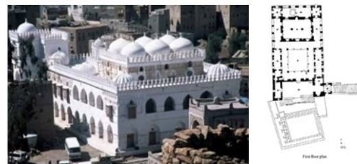
Figure 41. Plan and general view of sanctuary of the 'Amiriya Madrasa in Rada [30].
