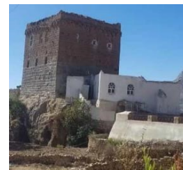
Figure 17. General view of the mosque from the Northern side.
