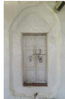
Figure 12. One of the mosque's windows with two wooden shutters.
