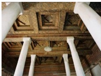
Figure 50. General view of muṣandqāt of the Al-Abbās Mosque. Source:[34]
