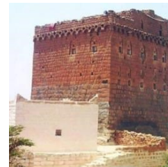
Figure 18. General view of the mosque before the recent additions on the southern side.
