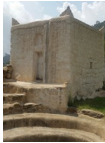
Figure 57. General view of 'aṭalha mosque. Source: photo of 'abdū Sa'd Al-Bīhīri
