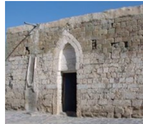
Figure 53. General view of Ṣarha mosque [35].
