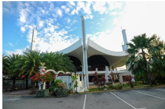
Figure 11. The building's front entrance of Seremban Mosque (Source: Author)
