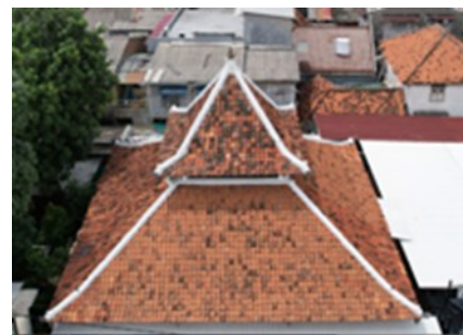
Figure 3. The Roof of Angke Mosque, (A) Mustoko, (B) Jurai
