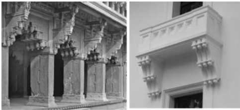
Figure 15. Detail of corbel Mughal Architecture (left) and Detail of Post Office Building (right), simplification (Author).
