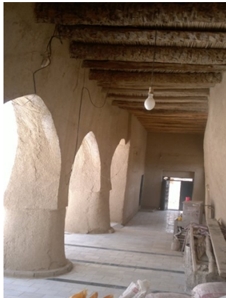
Figure 10. the entrance of the mosque and its corridor [28]
