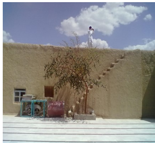
Figure 9. View of the central apron of the mosque [28]
