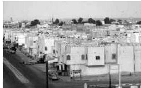
Figure 5. General view of 400 housing units in El Oued
