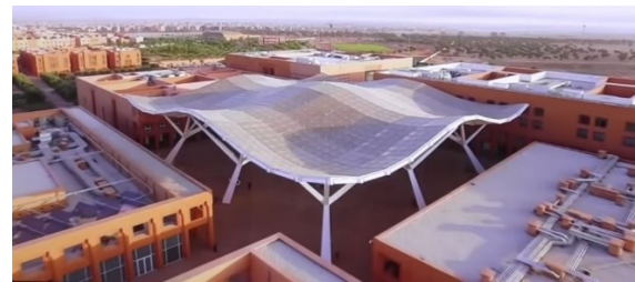
Figure 13. Urban Pergola, University design of integrated PV pergola and shade design. Source: Google image.
