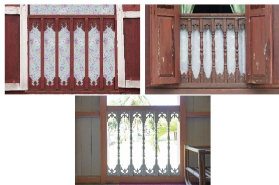
Figure 5. A total of 3 houses have six-piece panels with five columns on their window railing / jerejak tingkap .
