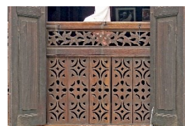
Figure 7. A total of one house has five-piece panels with horizontal panel on their window railing / jerejak tingkap .
