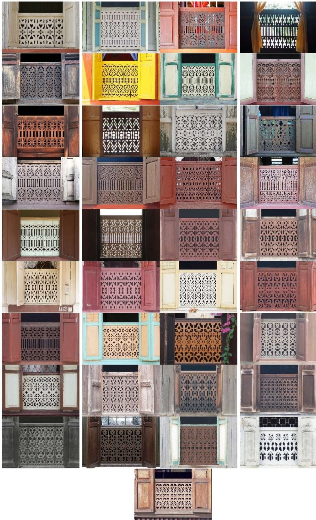
Figure 2. A total of 37 houses have five-piece panels on their window railing / jerejak tingkap.
