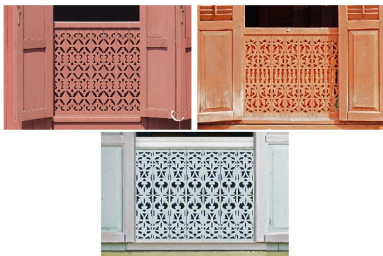
Figure 4. A total of 3 houses have seven-piece panels on their window railing / jerejak tingkap .
