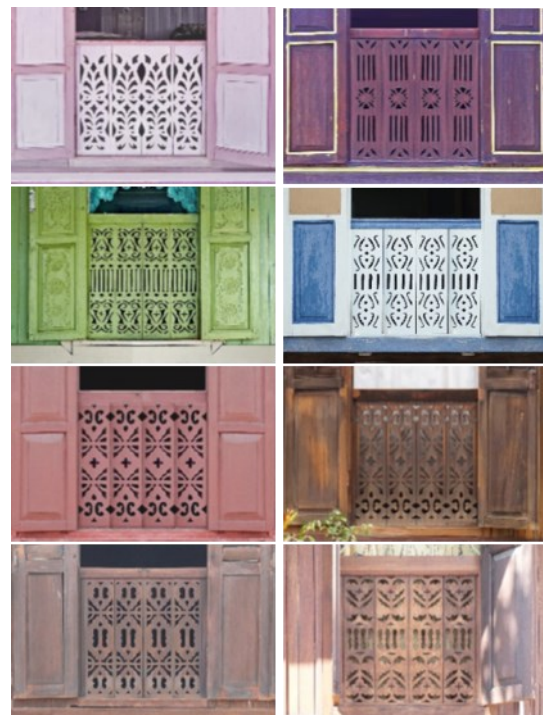
Figure 1. A total of 8 houses have four-piece panels on their window railing / jerejak tingkap ,
