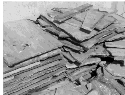
Figure 18. Original marble tiles as floor finishes being removed
