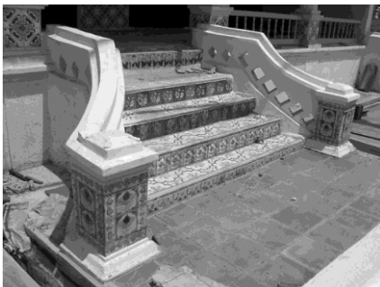
Figure 28. Stairs at the entrance of the mosque side
