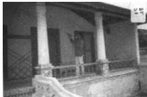
Figure 9. The Verandah; side view of Air Barok Village Mosque
