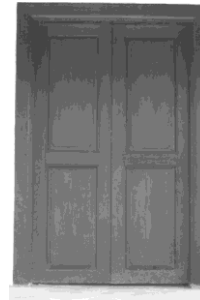
Figure 17. The detail of the window
