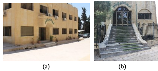
Figure 9. The administration building (Building 'B') entrances are not accessible: (a) the ground floor's entrance with two steps (Author); (b) The entrance of the first floor with many steps (Author)
