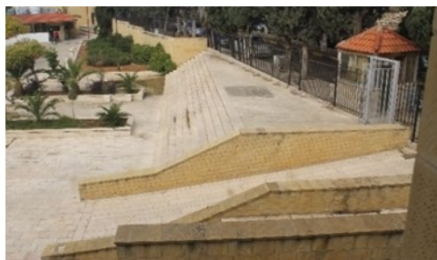
Figure 3. (a) Accessibility analysis of UJ Mosque's gates and entrances. The accessible entrance of building A is too far from the accessible community gate (Gate 1), Gate 2 has a steep ramp, and Gate 3 has stairs with no ramp (Author). (b) The ramp at Gate 2 does not follow standards, its height exceeding 75 cm (Author)
