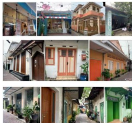
Figure 4: Building facade (source: survey, 2022)
