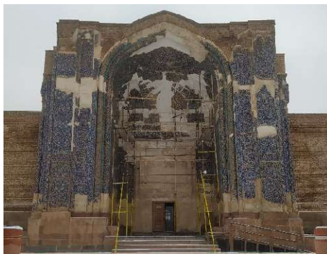
Figure 3. The entrance of the Mosque (North view) (Jan 2023)
