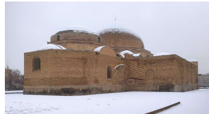
Figure 21. View from the southeast (Jan 2023)
