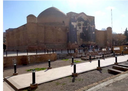
Figure 28. Northeast view of a mosque (Mar 2023)
