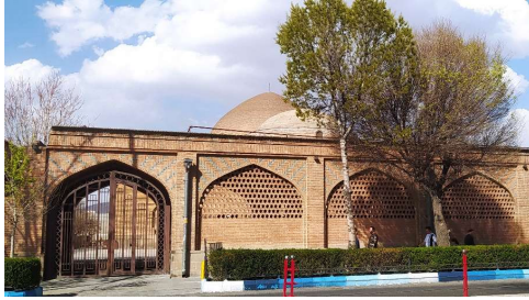
Figure 25. South view of the mosque from the Emam Khomeini (Pahlavi) street (Mar 2023)
