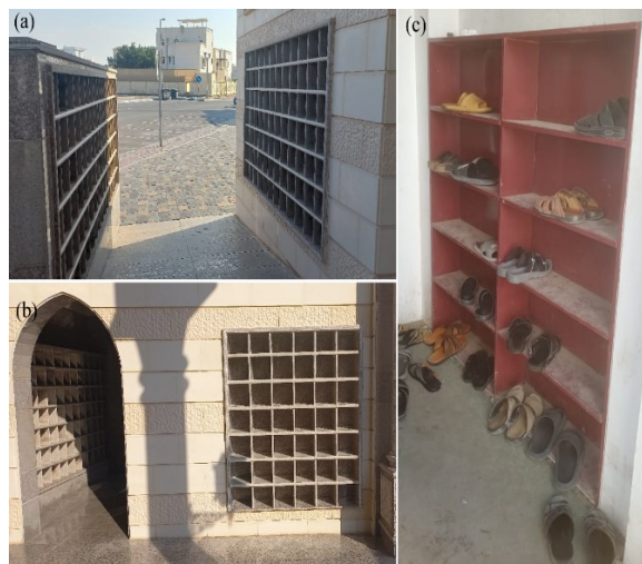
Figure 1 (a and b) Shoe racks in Sheikh Shakhboot bin Sultan mosque at Abu Dhabi. [Architect Rizwan Khan] (c) Image
