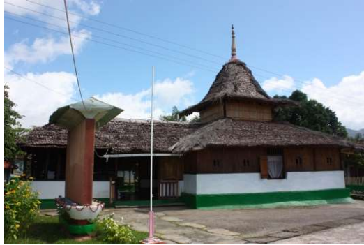
Figure 3. Two-tiered Roof Design
