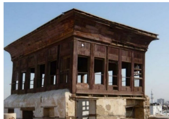
Figure 8. Use of a stairwell to distribute air inside the building rooms. MADY M., 2018, pp. 17
