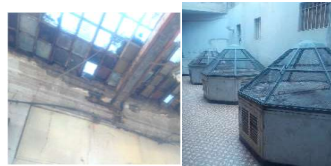
view of the Court
