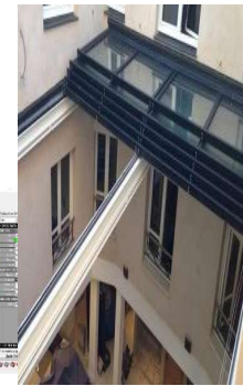
Mobile sliding roof canopy
