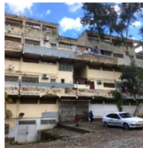
Small windows with brick guardrail
