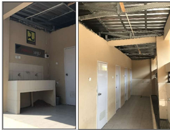
Figure 10. Communal shower and restroom at the Raudlatul Quran Islamic Boarding School
