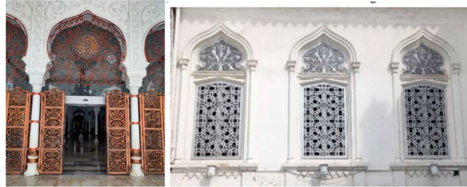
Figure 6. The door and the windows of the BGM [5]
