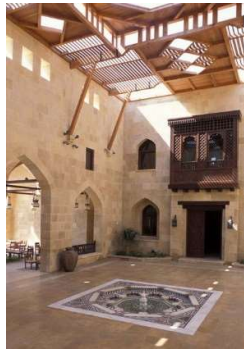
(a) Mashrabiya in the interior of the restaurant
