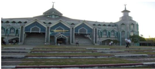
Figure 6. the Facade of Al Markas Al Islamic Makassar Mosque
