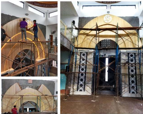
Figure 11. The mihrab construction process.
