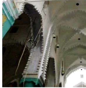
Figure 9. Keyed pendentive vaults (source: authors, 2024)
