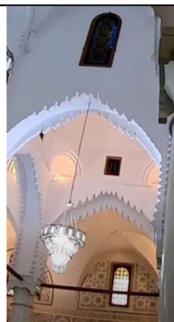
Figure 6. Arches with lambrequins (source: authors, 2024)
