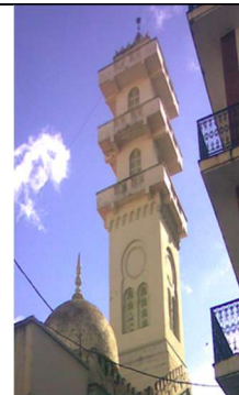
Figure 7. Square-section minaret (source: authors, 2017)
