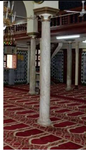
Figure 25. Marble columns (source: authors, 2024)
