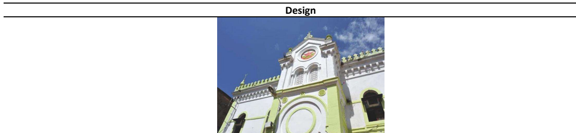
Figure 21. Entrance of Sidi El-Kettani mosque (source: authors, 2024)
