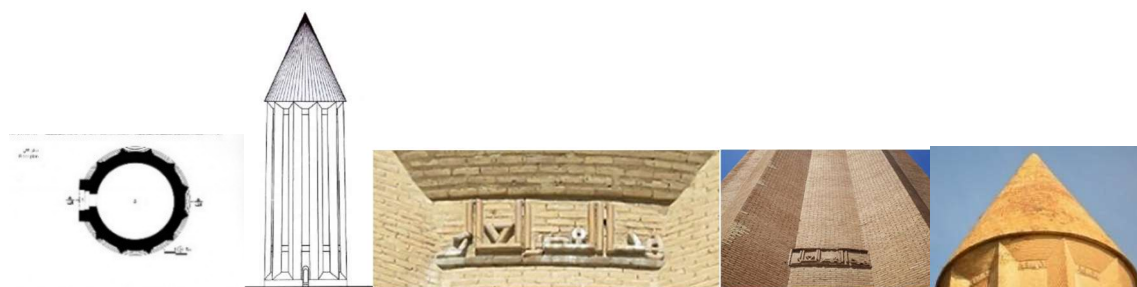
Figure 3. a: Decagonal Plan and Vertical Flanges. The 10-sided star-shaped base, created by radial flanges, highlights the tower's radial symmetry. b: Kufic Inscriptions. Horizontal bands of brickwork inscriptions commemorate Qabus ibn Wushmgir, emphasizing verticality and political symbolism. c: Brickwork Detail. Radial brick alignment along the flanges, showcasing Non-overlapped joints and structural stability.
