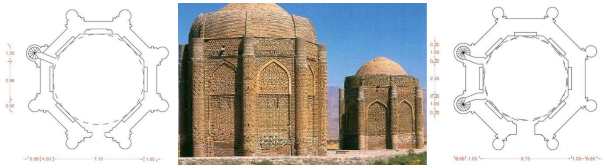
Figure 4. a. Kharāqan west (left) and East Tower (right), Qazvin, Iran. The octagonal monument has interwoven brick ribs and hybrid geometric patterns
