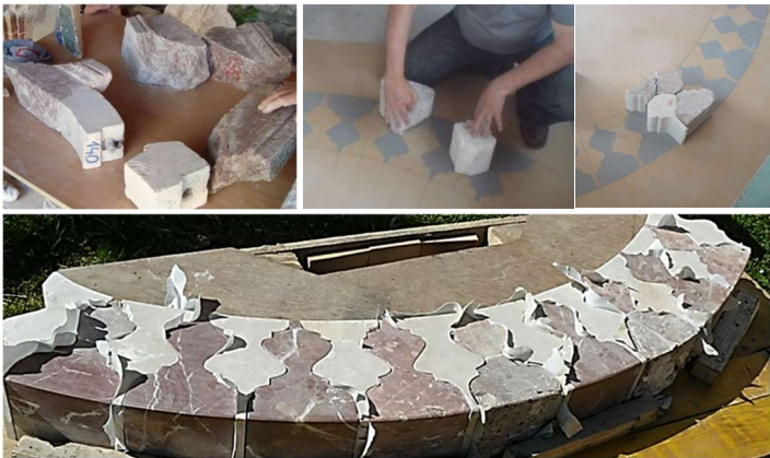
Figure 3. Making and preparing floral elements of the segmental arch of the mosque portal (A) (B) (C) (D)
