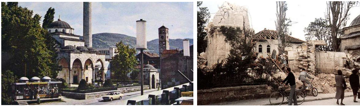
Figure 1. Ferhadija Mosque in Banja Luka, before and after war destruction (A) (B)
