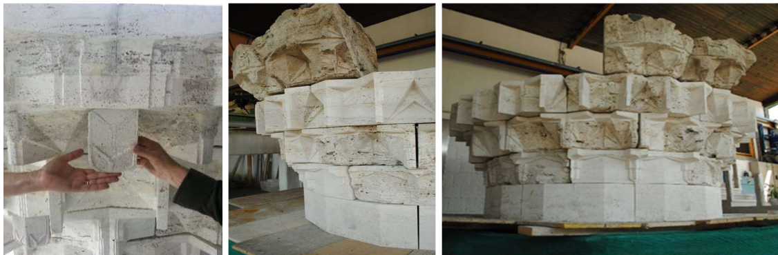
Figure 6. Şerefe parts in the workshop, assembling new and restored parts (A) (B) (C)
