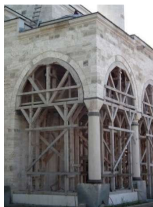
AFTER REHABILITATION FIGURE
