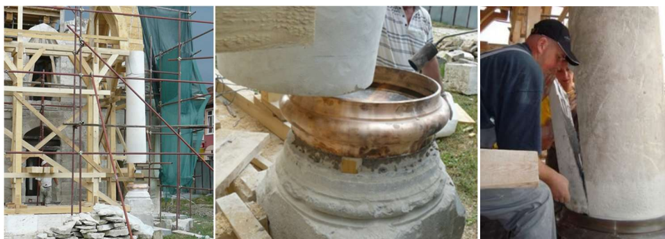
Figure 4. Installation of restored porch pillars (A) (B) (C)
