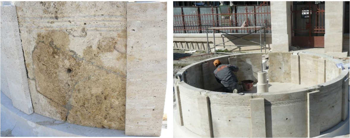
Figure 7. Restoration of one and reconstruction of the other elements of the fountain (A) (B)
