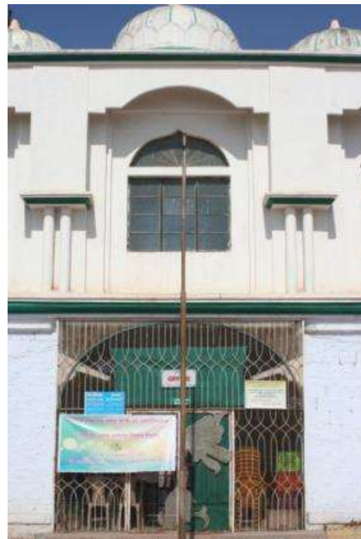
Figure 11. Gatehouse, with a few gallery chambers for guards. (Source: author, 2014)
