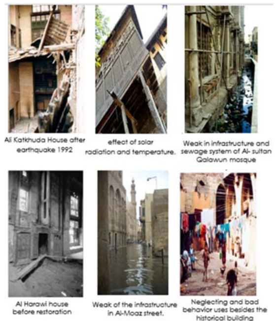
Figure 11. Forms of deterioration
