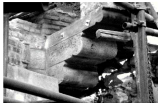
Figure 8. Wooden Corbel in Al-Razaz house1480 A.
