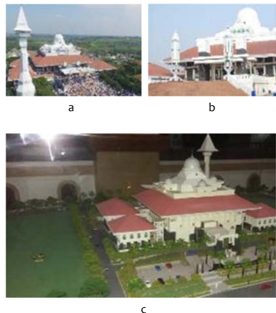
Figure 1. (a) Masjid Azzikra in Upper View [15] (b) Masjid Azzikra in Front View [16] (c) Masjid Azzikra Mock-up [17]
