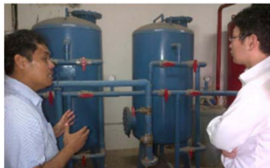
Figure 5. Recycling Water System from Used Ablution Water [21]
