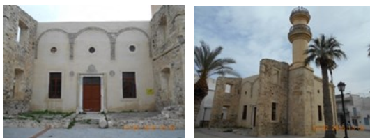
Fig. 10: Ierapetra Mosque, the minaret, and the portico's traces Fig. 11: the portico and the prayer hall's main façade
