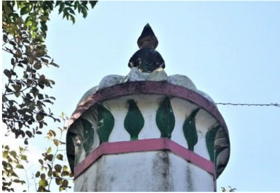
Figure 14. Corner turret & cupola, (photograph by Authors)
