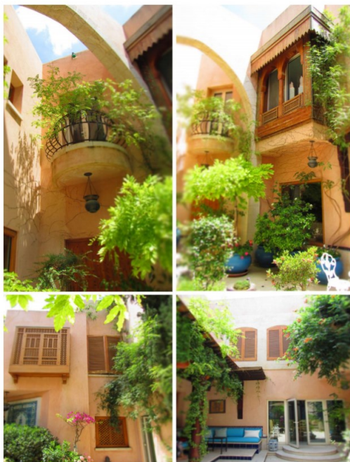
Figure 25. The courtyard entrance arch (top left); the Mandalon (top right); the Mashrabiya (bottom left); and the wooden louvered windows (bottom right). [Source: the author]
