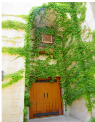
Figure 10. The house Iwan has a door and a Mashrabiya above [Source: the author]
