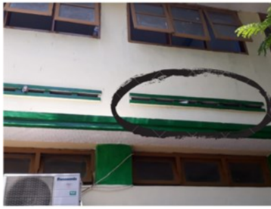
Figure 5. The lower ventilation in the classroom (Source: the author)
