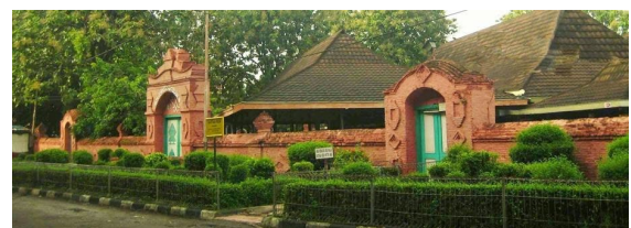
Figure 16. The Enclosure of Sang Cipta Rasa Mosque [12]
