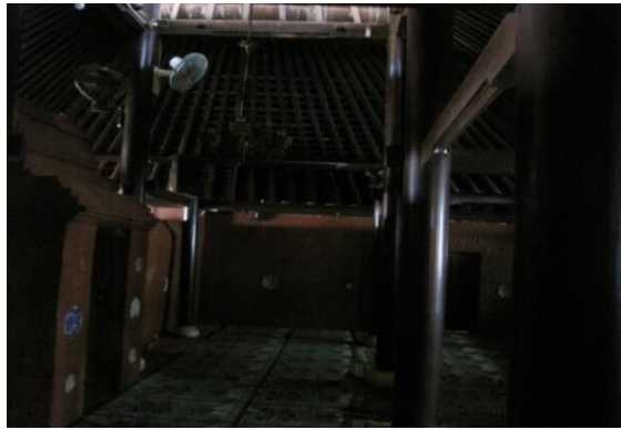
Figure 12. Panjunan Red Mosque Sakaguru [11]
