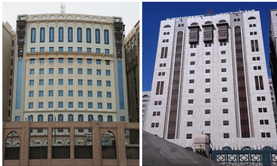
Figure 5: Other examples of the false Rowshan in the Central District show the discrepancy between the size of Rowshan and the façade of the building. It is also noted that Rowshan's place on the top floors indicates that Rowshan was added to the building without any study or minimal knowledge of its basic functions.
