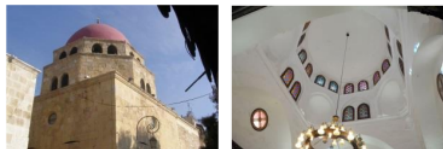
A. The dome from the outside
