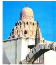
A. The dome from the outside
