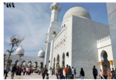
Figure 4. Sheikh Zayed Mosque - Front View
