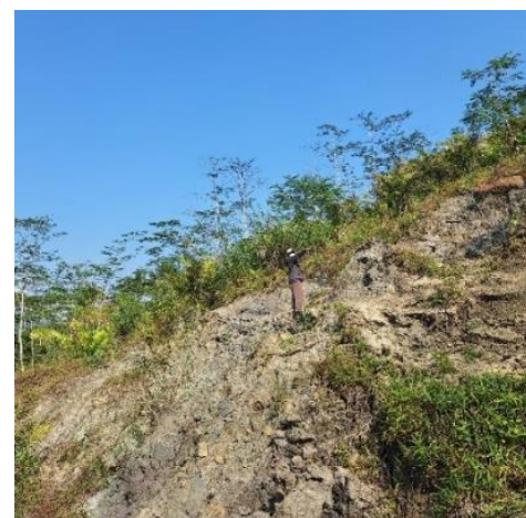
Figure 6. Landslide Location at Point T5
