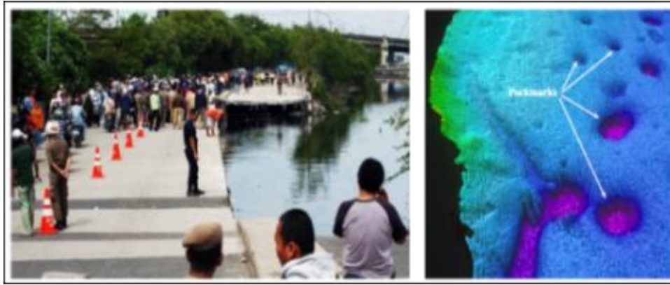
Figure 1. Left: Subsidence at Jl. R.E. Martadinata (North Jakarta), September 2010; 6 Right: Pockmark caused by subsidence 7
