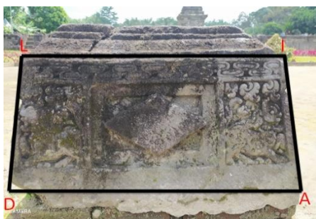
Figure 5a. Umpak Left Side View
