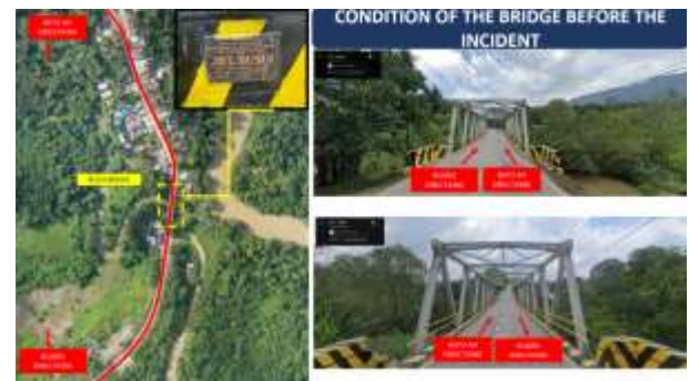
Figure 2. Condition of the bridge before the incident
