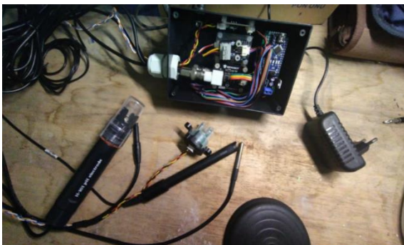
Fig 15 Installation of all sensor cables to each sensor module
