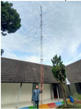
Figure 9. The Main Author beside antenna tower for network infrastructure inspection.
